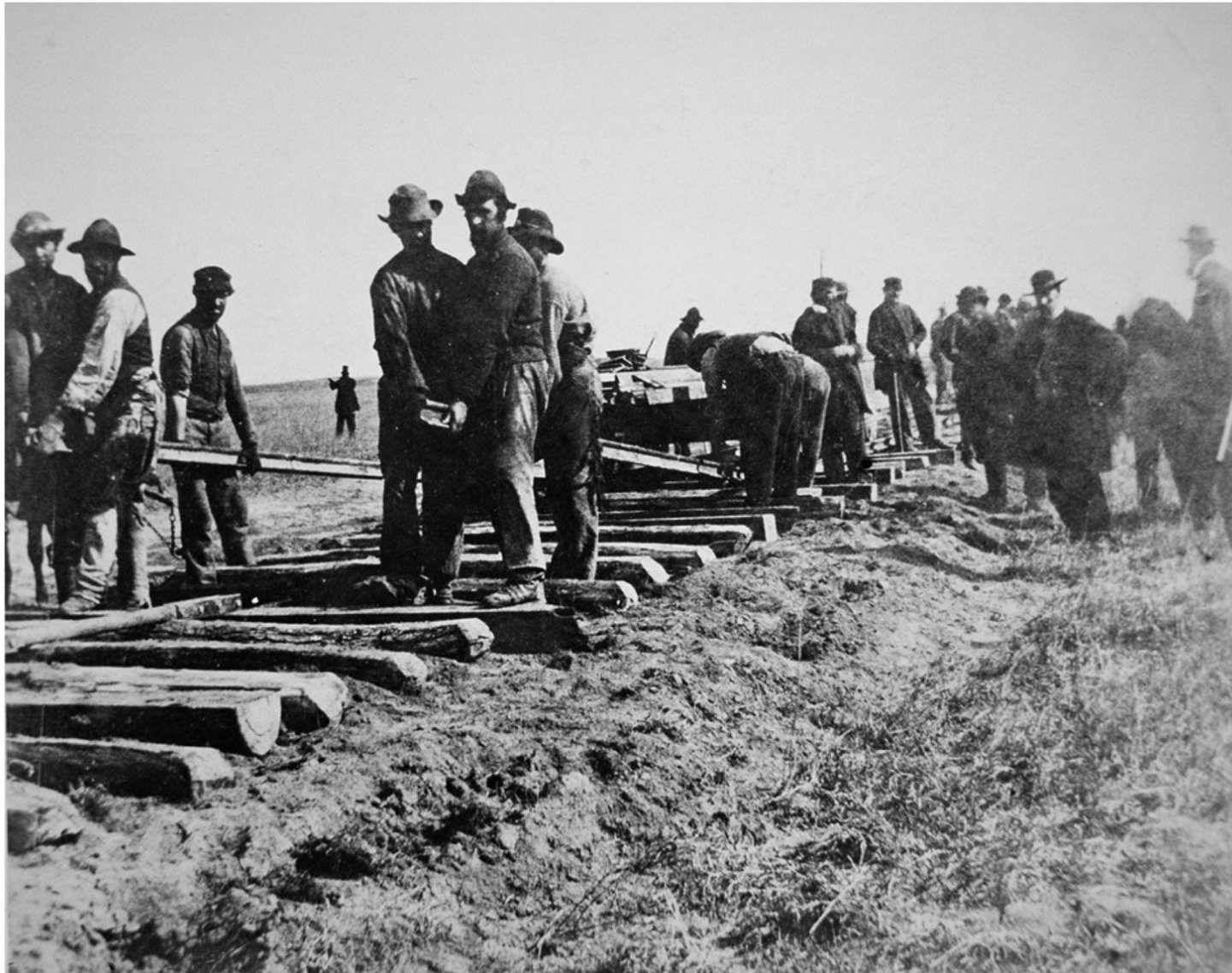
Track-layers gang-building the Union Pacific Railroad through American wilderness, 1860s, (b/w photo), American Photographer, (19th century)/Private Collection, Peter Newark American Pictures/The Bridgeman Art Library
